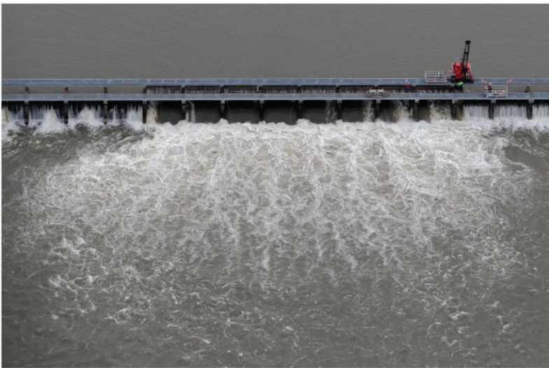
Workers open bays of the Bonnet Carre Spillway, to divert rising water from the Mississippi River to Lake Pontchartrain, upriver from New Orleans, in Norco, La., on May 10, 2019. Gerald Herbert—AP
